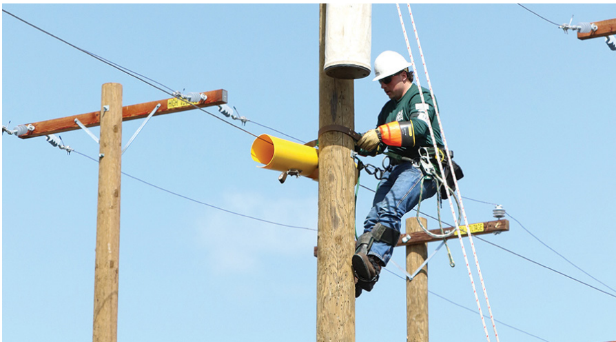
Members of the Owatonna Public Utilities team place the cover up in preparation for changing out the crossarm under energized conditions.
