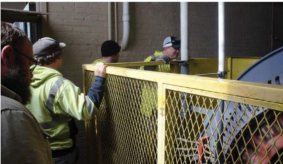
Students examine a generator up-close at the Brainerd hydro dam.
